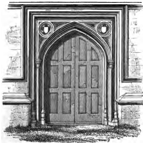
155. Fotheringhay, Northamptonshire, A.D. 1440.
